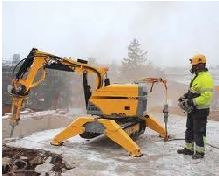
On the yard
